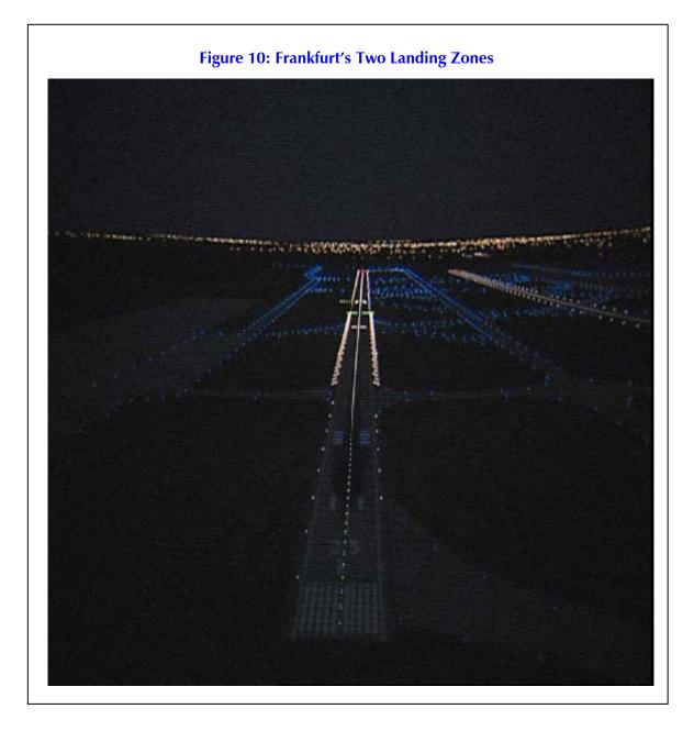
This represents the displaced threshold being lit and the beginning portion of the runway unlit so that the arriving aicraft is directed to displaced portion for landing. (Source: Frankfurt Airport Capacity Enhancement Program the Role of Wake Vortex Reducing Measures 2nd WakeNet 2 - Europe Workshop, 30.11. – 01.12.2004)
