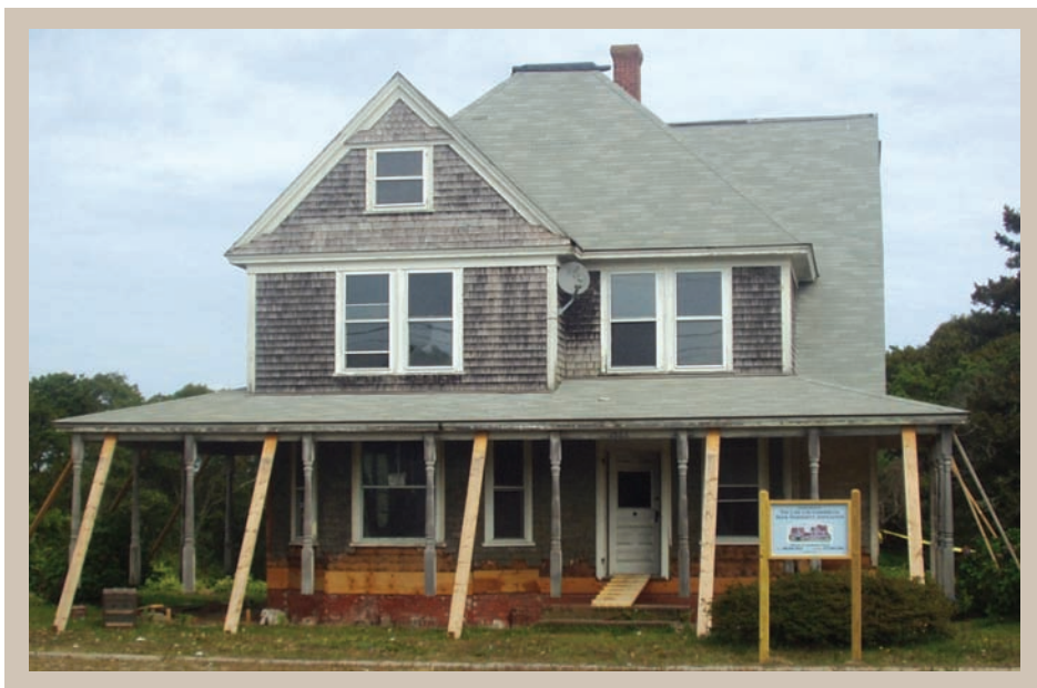
Captain Harding House under renovation.
