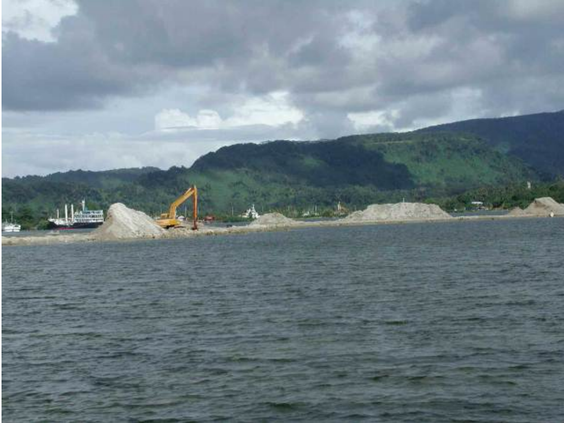
Figure 15. Massive dredging near Sokehs Rock, an important tourist spot in Pohnpei. The dig is to complete a new airport extension to bring in more tourists. A lack of environmental control allows sedimentation plumes to spread throughout the lagoon near Sokehs following Pohnpei's infamous rains (Photo: K. Rhodes, February 2010)
