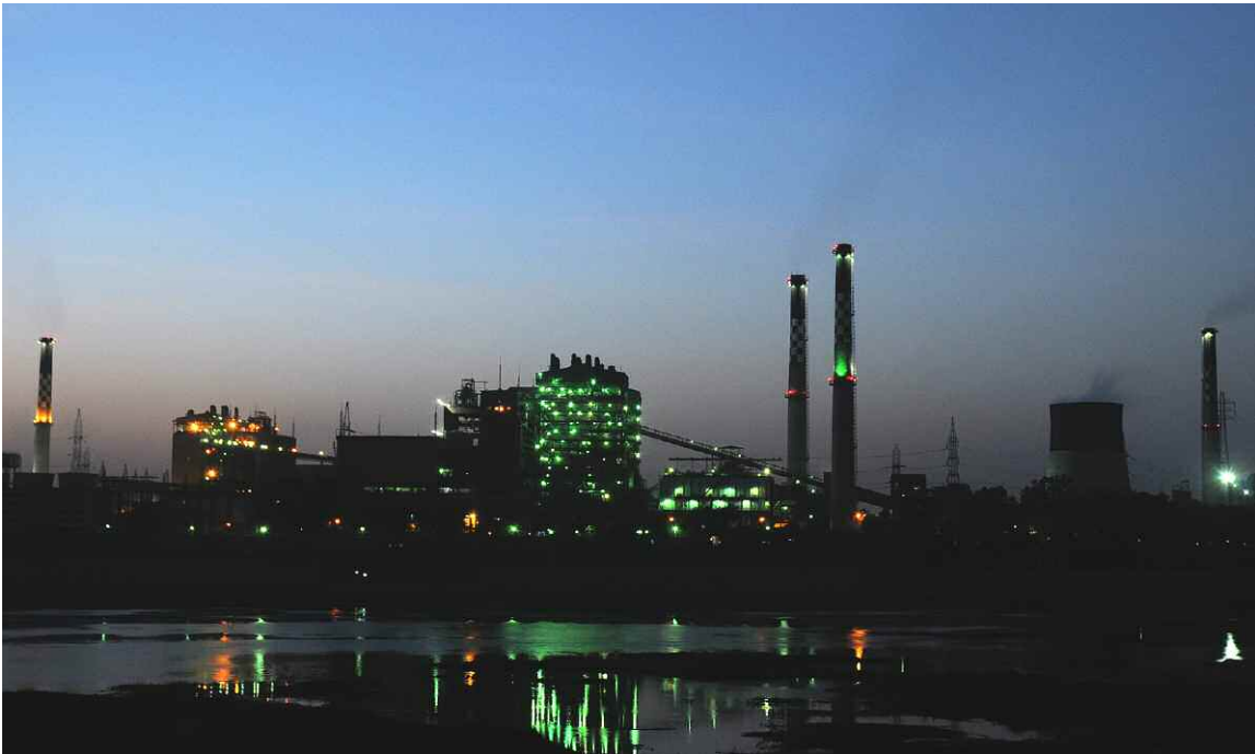
Sabarmati Thermal Power Station, which powers the Indian cities of Ahmedabad and Gandhinagar (Photo credit: Koshy Koshy)
