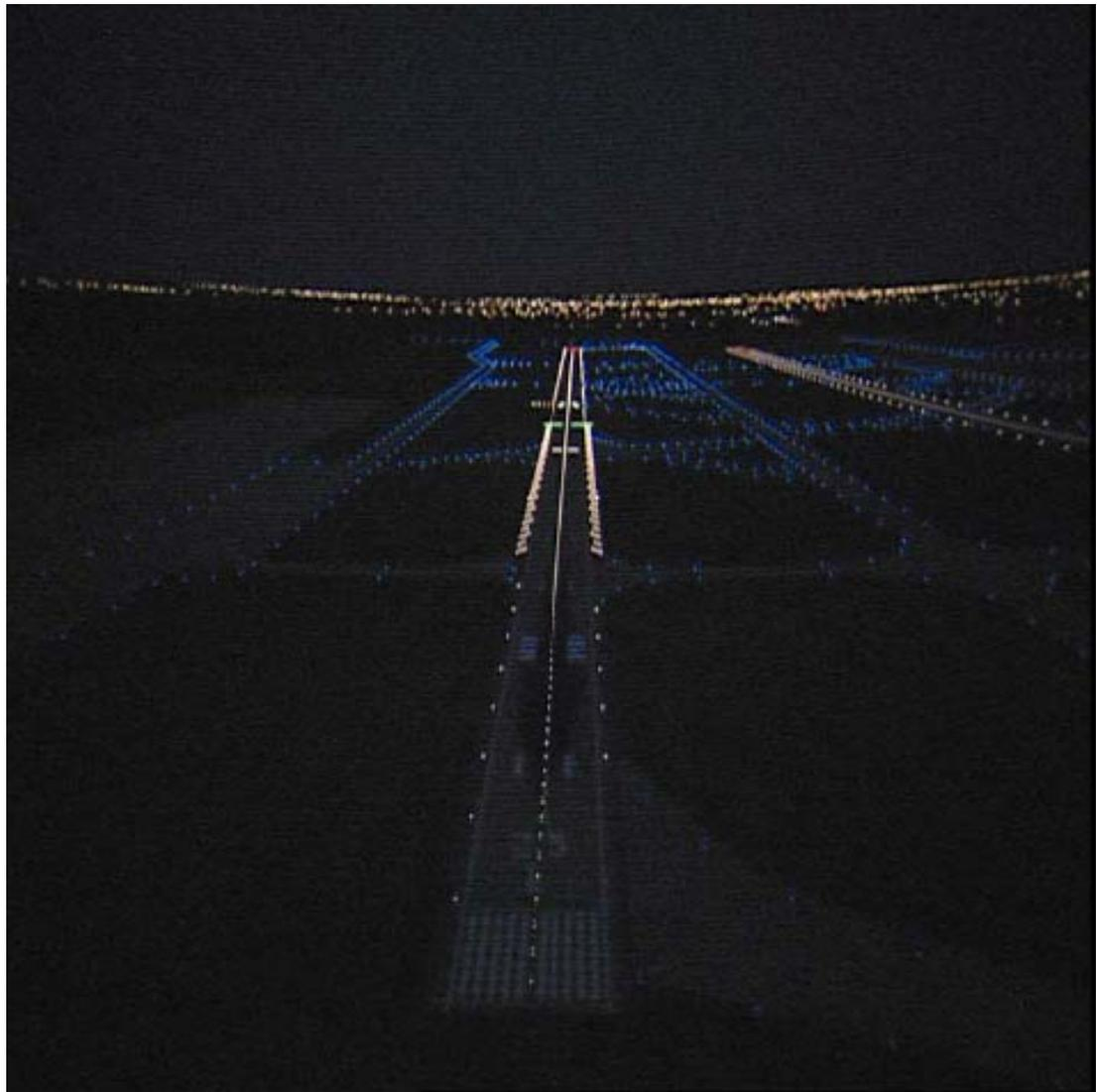
*This represents the displaced threshold being lit and the beginning portion of the runway unlit so that the arriving aircraft is directed to displaced portion for landing. (Source: Frankfurt Airport Capacity Enhancement Program the Role of Wake Vortex Reducing Measures 2nd WakeNet 2 - Europe Workshop, 30.11. – 01.12.2004)*
