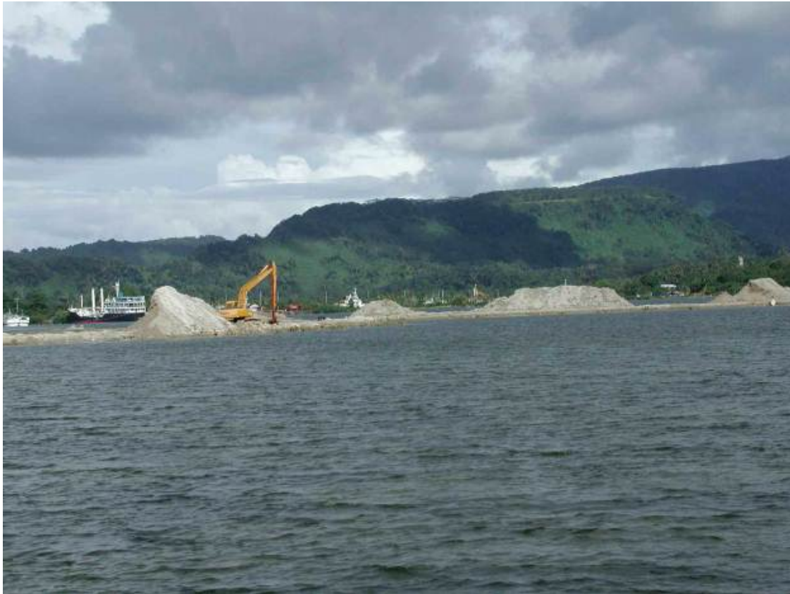
Figure 15. Massive dredging near Sokehs Rock, an important tourist spot in Pohnpei. The dig is to complete a new airport extension to bring in more tourists. A lack of environmental control allows sedimentation plumes to spread throughout the lagoon near Sokehs following Pohnpei's infamous rains (Photo: K. Rhodes, February 2010)
